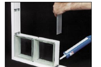
Silicone sealant is applied to vertical and horizontal aluminum spacers that intersect and bond metal to blocks, without mortar.
