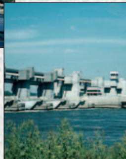
Lock and Dam
